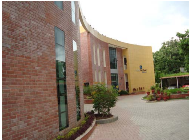
Manufacturing plant of Rotomag in Anand, Gujarat
