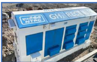
2x558kW Containerised Rectifiers - 3600A/ 155V for NTPC, Leh Green Hydrogen Mobility Pilot Project (Forced Air-Cooled; Outdoor Container Type)
