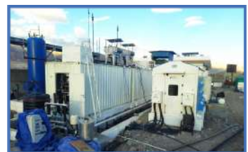
2x558kW Containerised Rectifiers - 3600A/ 155V for NTPC, Leh Green Hydrogen Mobility Pilot Project (Forced Air-Cooled; Outdoor Container Type)
